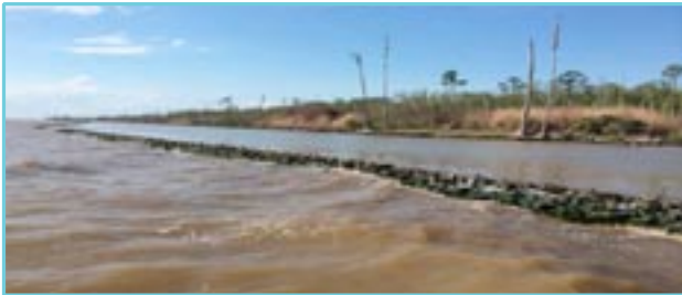
Breakwaters on Mobile Bay protect the shoreline from erosive wave energy. Photo courtesy of The Nature Conservancy
